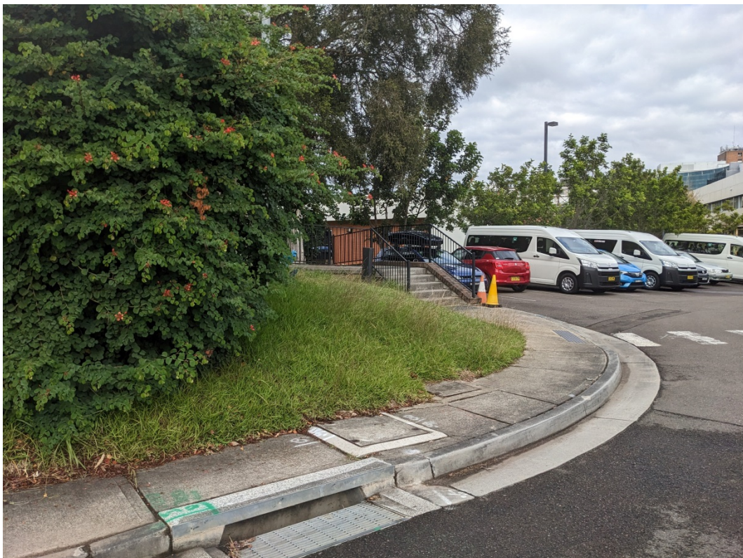
Photograph 2: View of pedestrian and stairs
