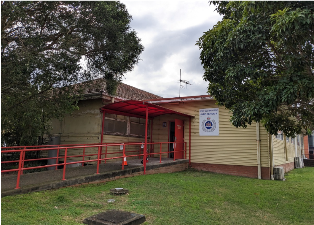
Photograph 3: View of the fire service building
