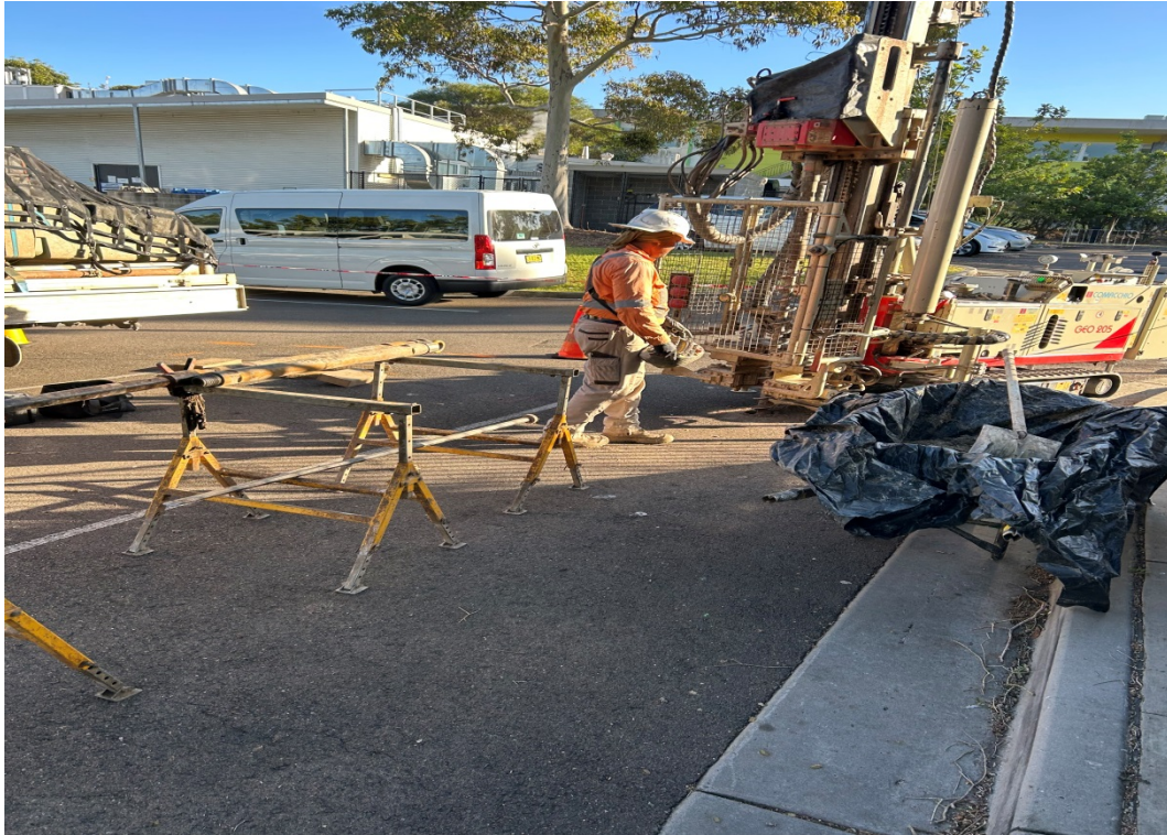
Photograph 1: View of drilling at the car park
