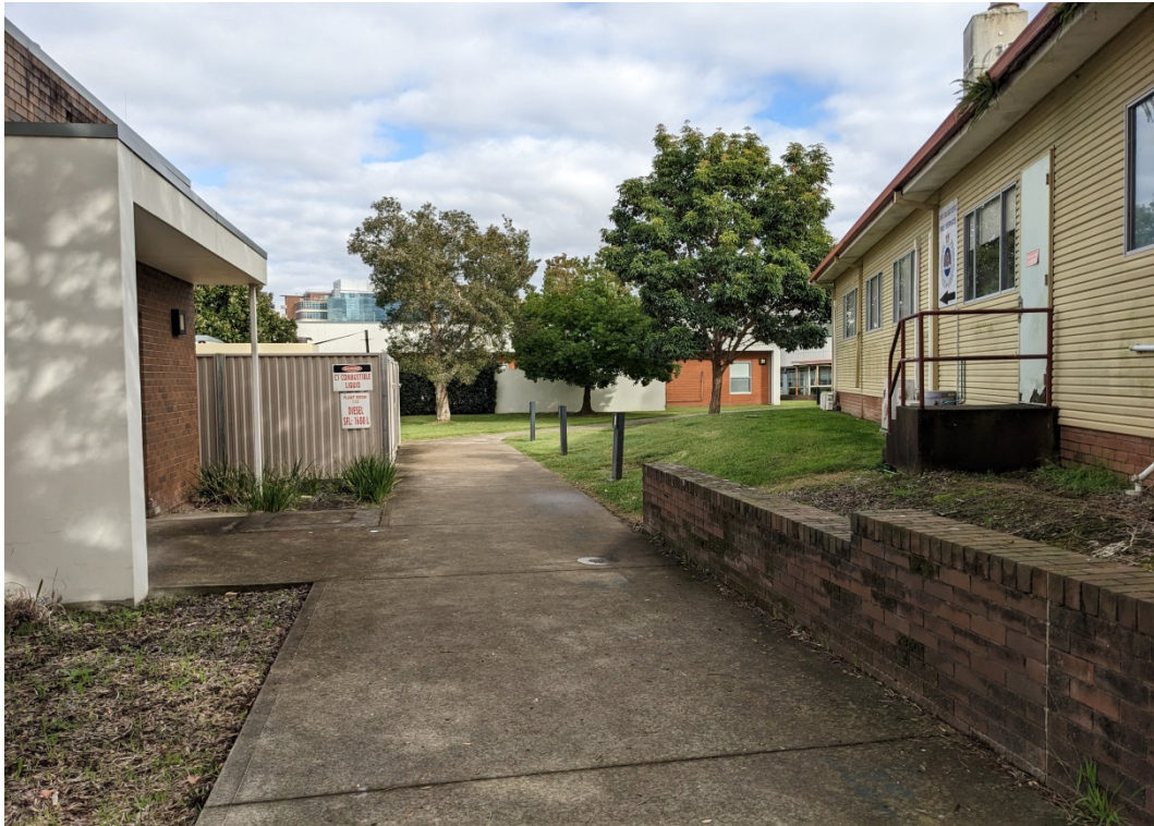
Photograph 5: view of the footpath at the other side of the building.
